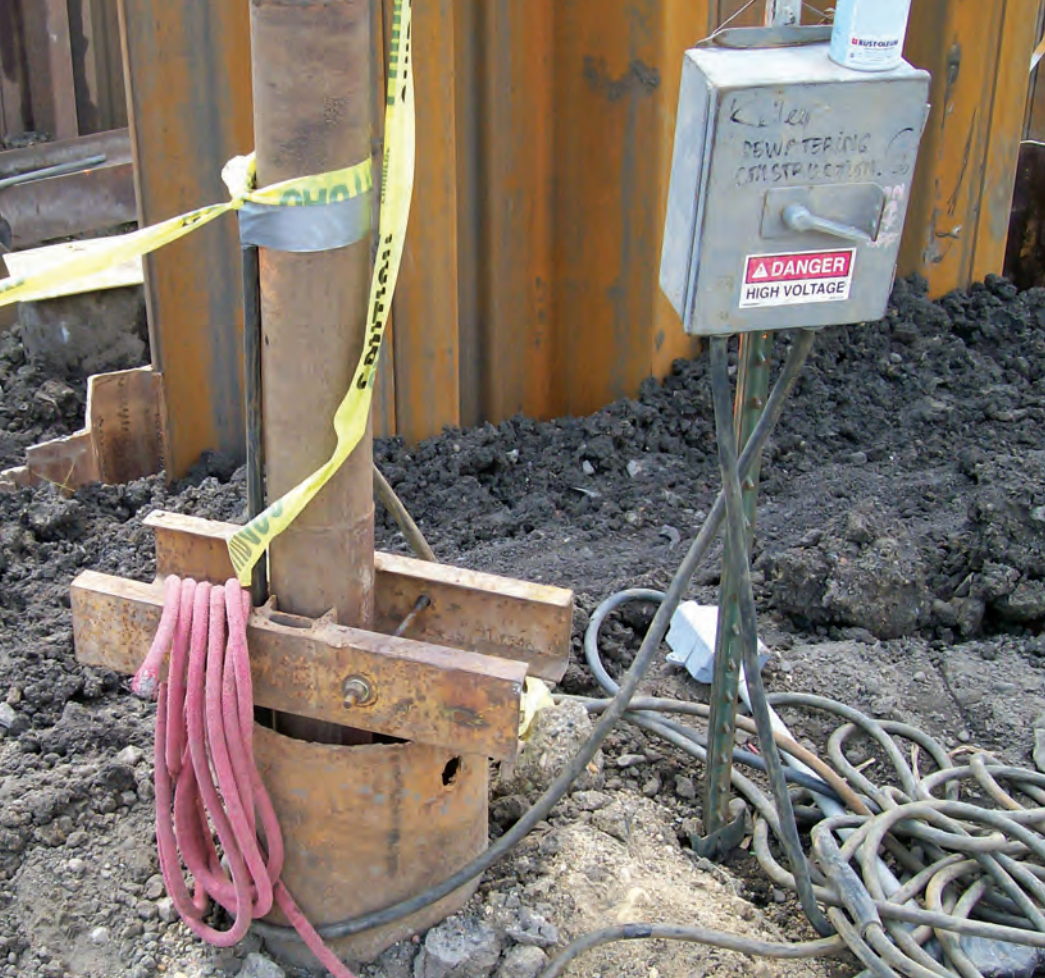
One of the dewatering wells recently installed.
