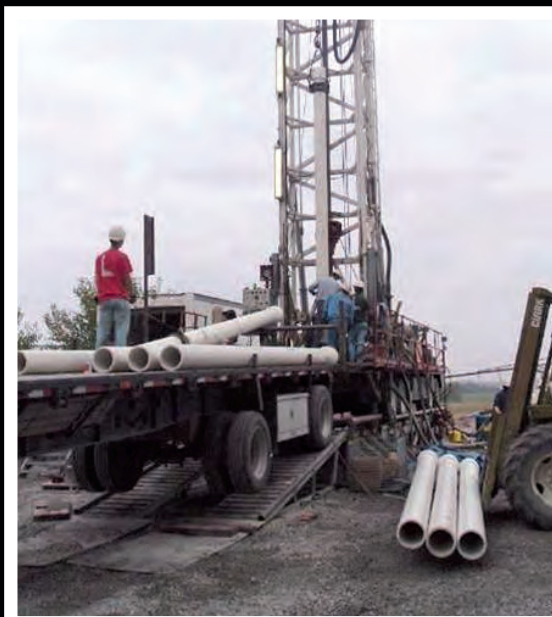
FIGURE 2. Installing casing.
